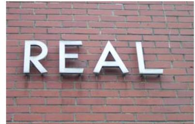
**Not Recommended:** Positive cut out letters on historic masonry. Installation will damage the building material.
