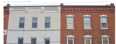
**Not Recommended: Covering original exterior materials.** The covering with stucco of the exterior brick of one of the buildings in a row of similar buildings damaged the historic architectural integrity not only of the specific building, but of the entire streetscape.
