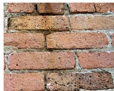
**Not Recommended: Sandblasting masonry.** These sand-blasted bricks are pitted and eroded. They lack their outer protective surface.
