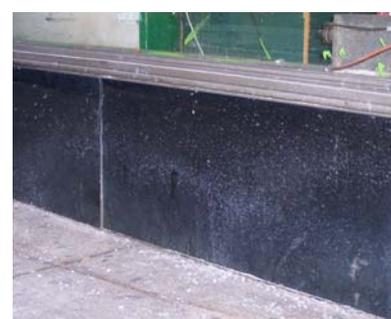
**Recommended: Preserve pigmented structural glass.** This material was frequently used below display windows for bulkheads.
