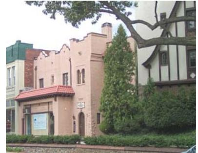
**Recommended: Retain original historic materials.** A variety of exterior wall and roofing surfaces distinguish the District's buildings. The stucco, stucco and half-timbering, bricks, and clay tile materials are among historic building materials that should be retained and repaired on these buildings along Garber Square.
