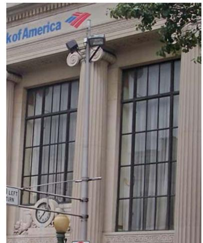
**Recommended: Preserve original window sash.** The bank at 56 East Ridgewood retains the multi-paned metal windows installed when the building was erected in 1930.
