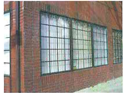
This new storefront has a sense of enframement and the 3-part division with bulkhead, large display window, and frieze. The division of the window into multiple panes would not be appropriate in most District locations.
