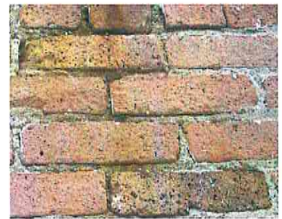
Not Recommended: Sandblasting masonry. These sand-blasted bricks are pitted and eroded. They lack their outer protective surface.
