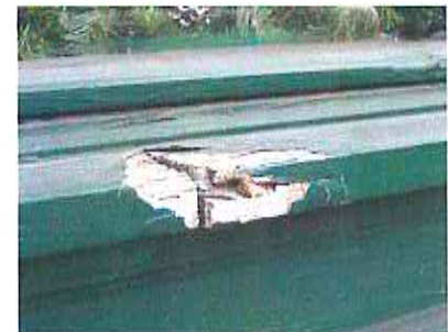
Recommended: Repair only the damaged section of historic wood features. This sill can probably be repaired with epoxy fill and then caulked. After repair, the entire element should be repainted.
