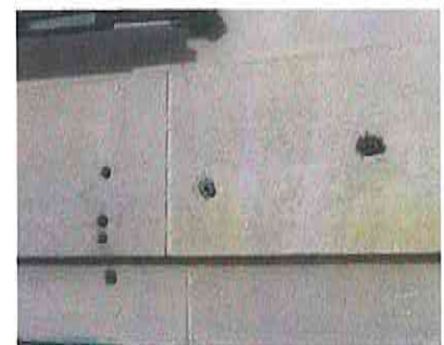
Not Recommended: Drilling holes in historic masonry. These holes remain although the signs and other attachments are gone.
