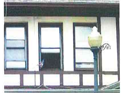
Recommended: Repair or renew historic stucco and wood. Half-timbering on buildings in the District combines stucco and applied wooden members.
