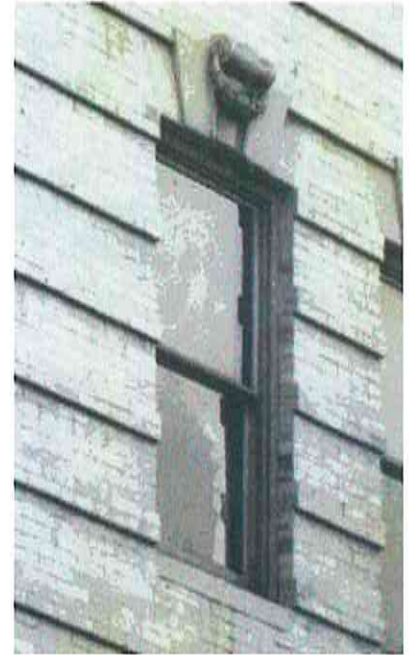
Recommended: Preserve historic upper-story windows. This early photograph shows a window with typical 1/1 double-hung sash.
