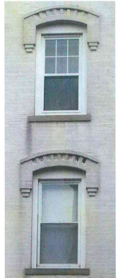
Not Recommended: Using sash with inappropriate division of panes. The upper-sash with new 6/1 sash does not match with the lower 1/1 sash.
