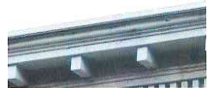
Recommended: Maintain and preserve historic exterior building materials. Cornices may have wooden elements, but frequently other materials are also used. Here the decorative frieze is painted brick.
