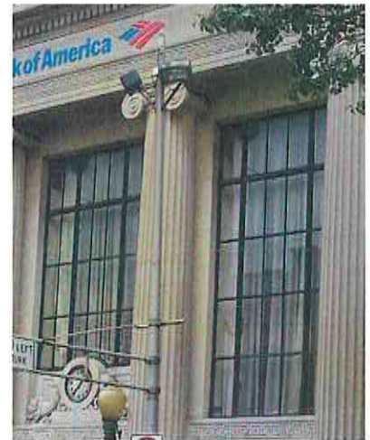
Recommended: Preserve original window sash. The bank at 56 East Ridgewood retains the multi-paned metal windows installed when the building was erected in 1930.
