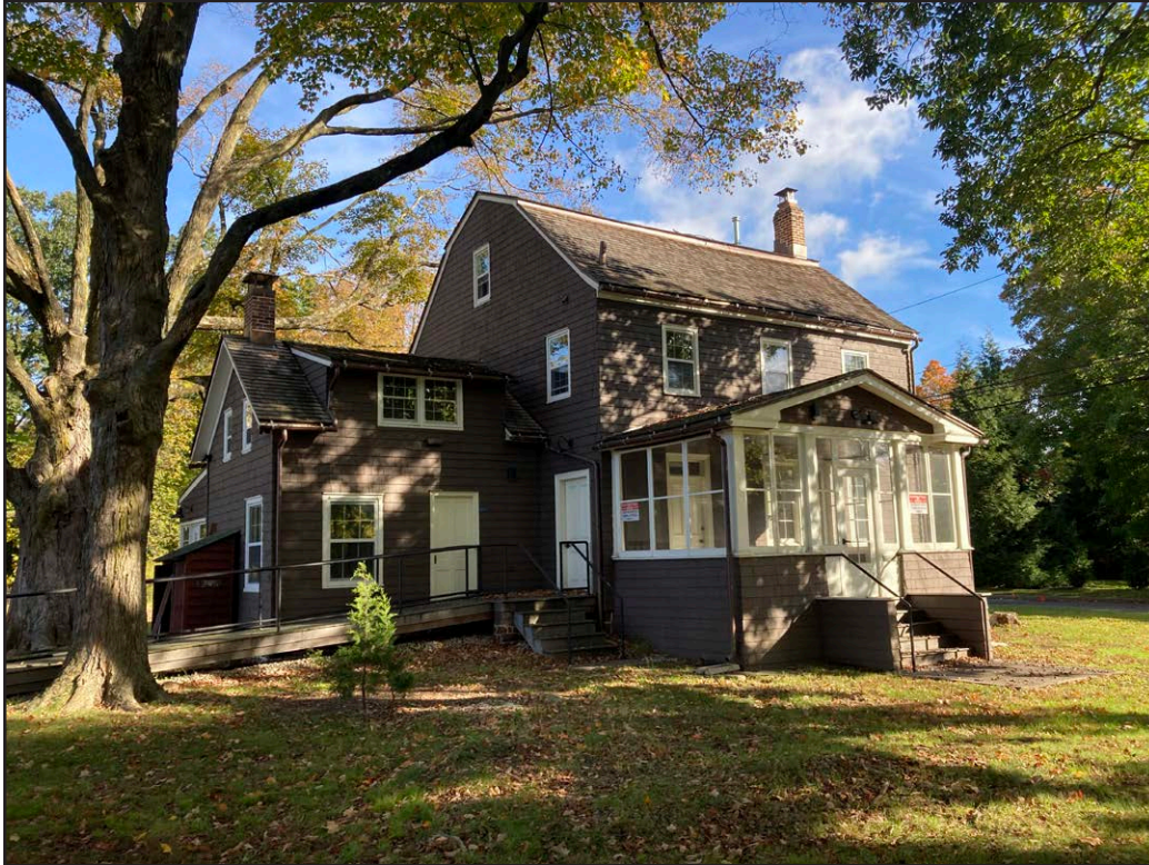
Plate 4.1: View of the John A. L. Zabriskie House showing the south (front) and west elevations.
