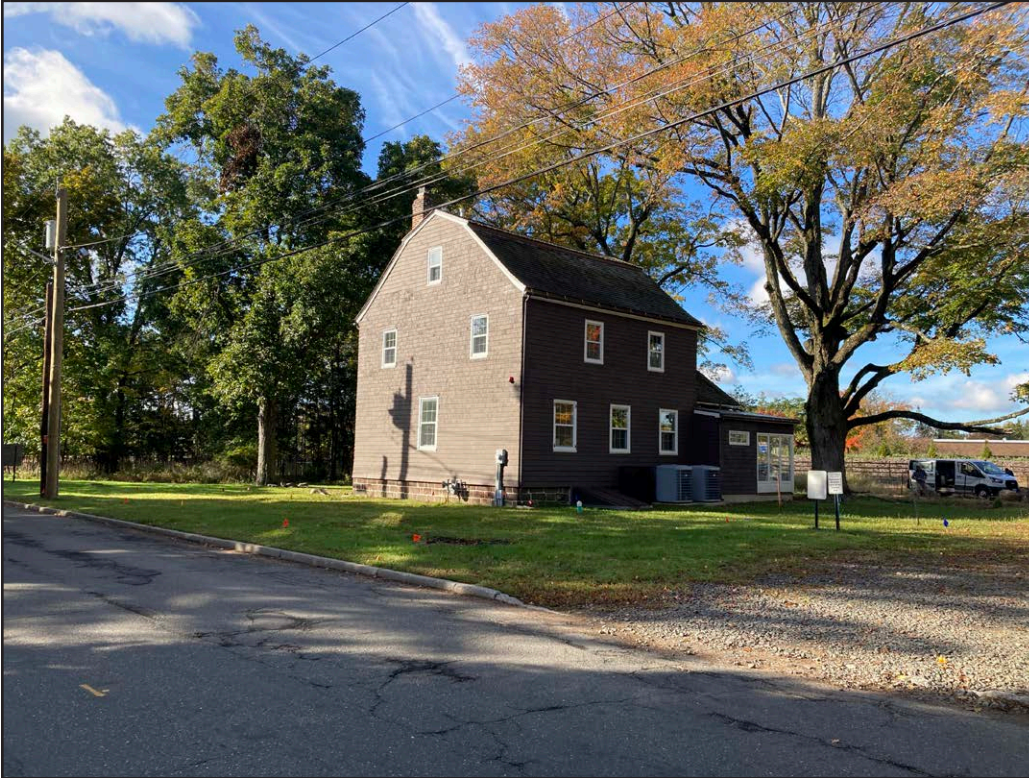
Plate 4.3: View of the John A. L. Zabriskie House showing the north and east elevations from West Saddle River Road.
