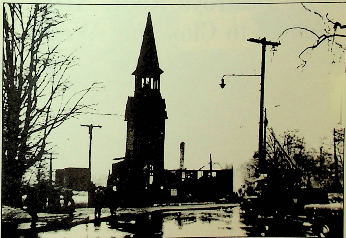
This is what was left of the First Reformed Church the morning after the fire. Because of its unstable condition, the steeple had to be knocked down by a crane.
