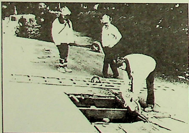
Firemen practice "opening up a roof" of a fire building to vent smoke and hot gases. This enables other firefighters to enter rooms below with a hose line to safely and quickly extinguish the fire. It also helps to limit the spread of flames and affords occupants a better chance of survival. Pictured left to right are: Capt. Albert Whitaker, Capt. Robert Thomsen, and Lt. Mark Bombace.
