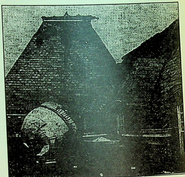
The steel covered cupola lies on the second floor roof after toppling off the gutted tower. Firemen were kept away from this area for fear that the cupola would fall while they were fighting the blaze.
